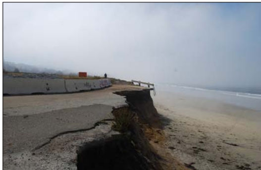
Erosion destroyed old roadways through El Granada and continues to move toward Highway 1.
