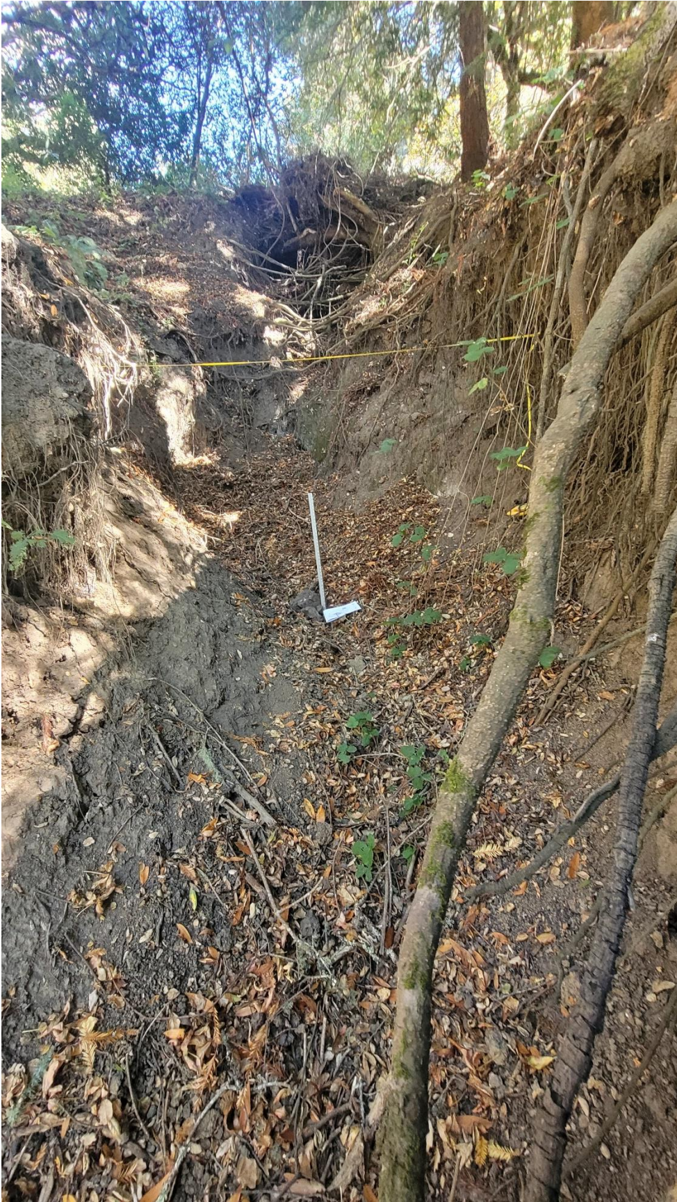
Photo 3: Erosion on parcel 078-120-060 from runoff of abandoned culvert that previously directed the flow of water from the culvert in photo 1. Damaged area measures approximately 45' long x 10' wide x 7' high.
