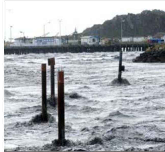
2011 – JAPAN tsunami in Crescent City, strong currents ripped piers apart. It may not look dramatic, but these currents lasted for days and were strong enough to destroy the harbor.
