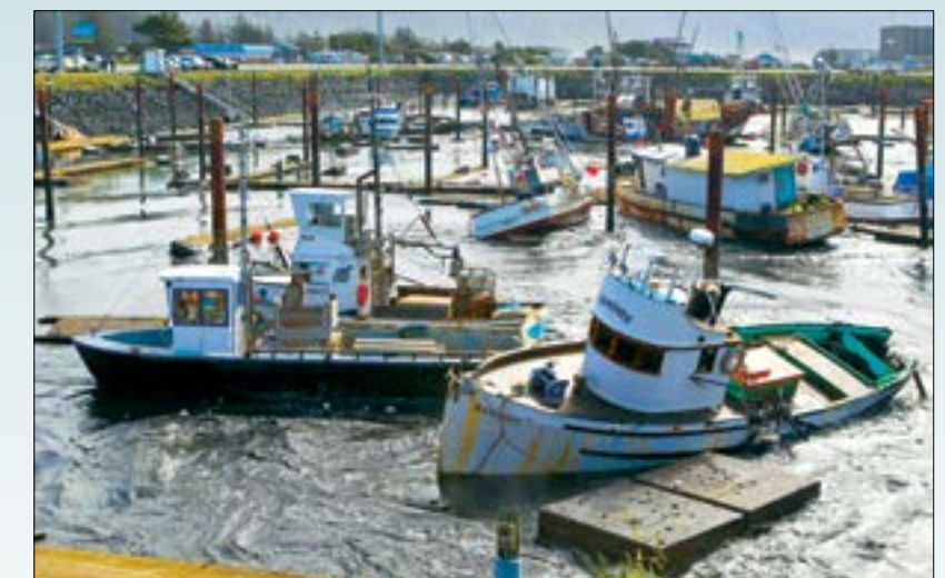
All the damage to Crescent City' Harbor's small boat basin was caused by strong currents and occurred more than two hours after the first tsunami wave arrived.
