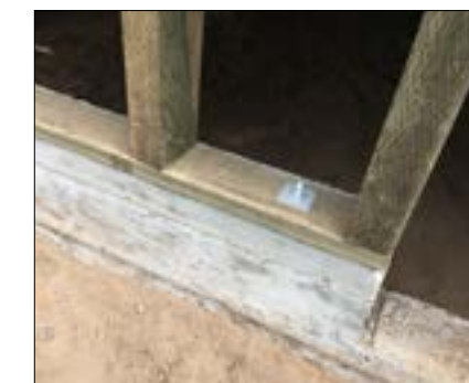
House bolted to foundation
