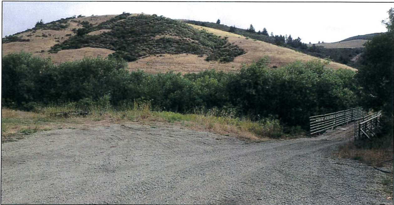
The developed/disturbed habitats on the south side of the existing railcar bridge. View facing north. Photo taken on July 12, 2016.
