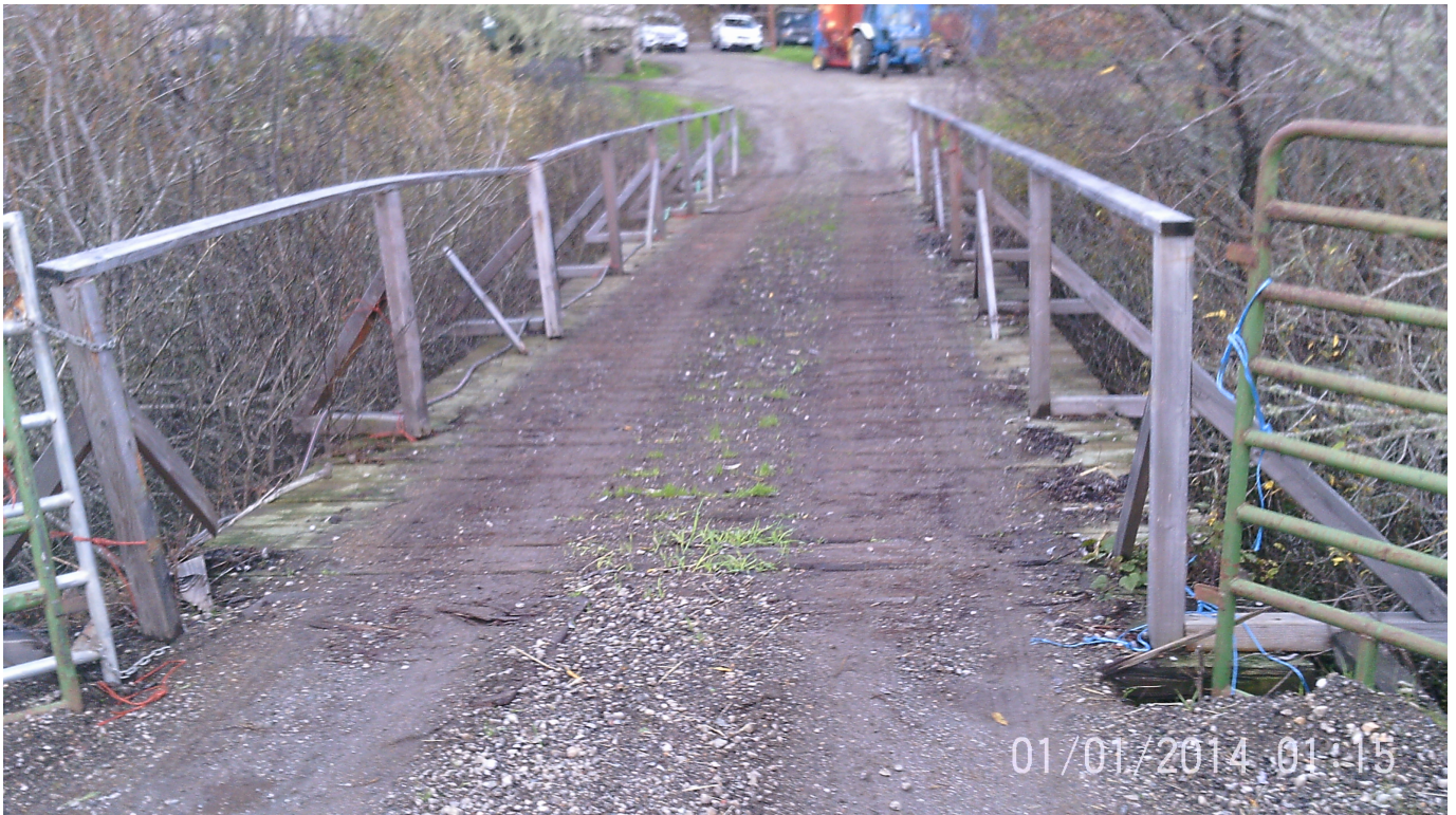
Existing Bridge, View South
