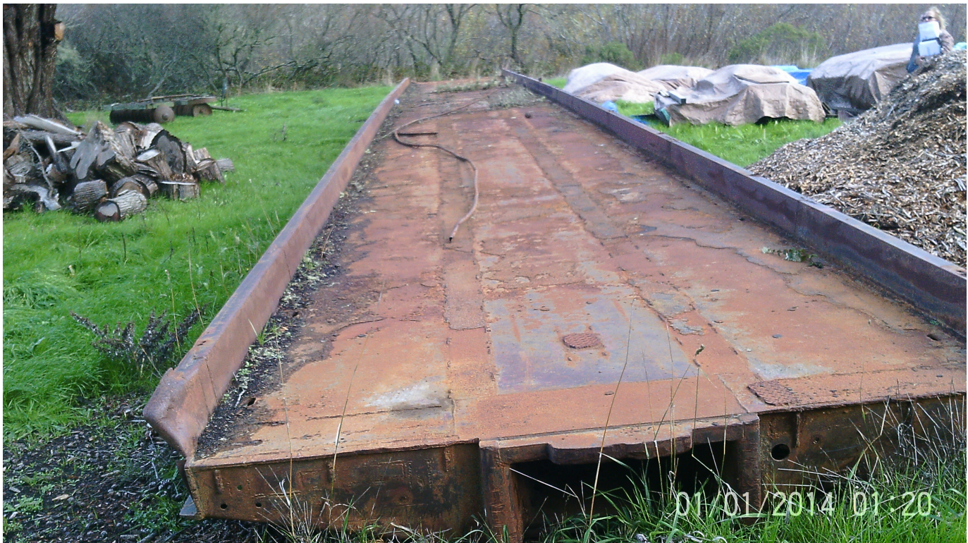
New Railcar Bridge For Expansion
