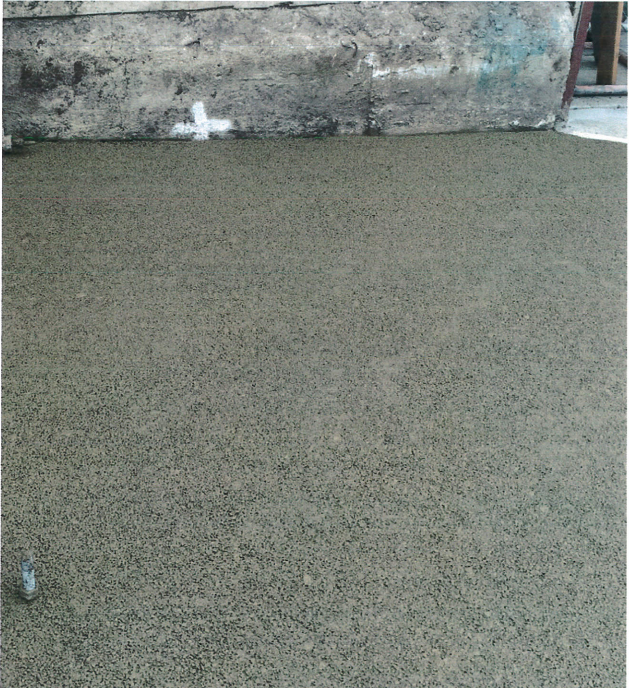
Figure 2. Porous Concrete Paving (typical)
